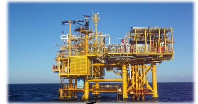
Existing Oyong pipeline to shore
