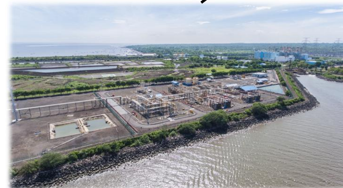
Existing Grati gas processing facility
